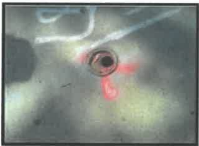
Water Gate Valve
